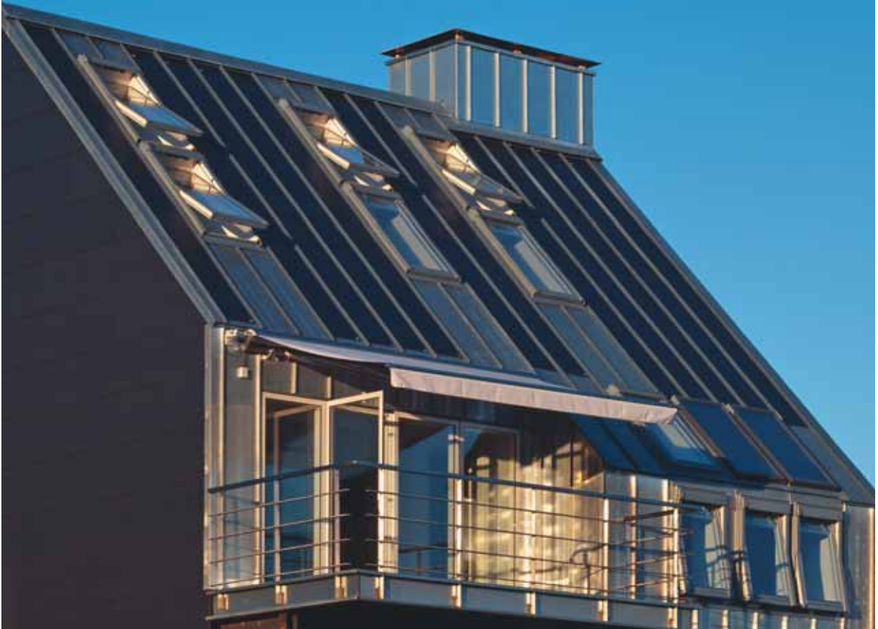
SOLTAG, A NEW WAY OF CREATING A SYNTHESIS OF ARCHITECTURE, DAYLIGHT AND ENERGY. PREFABRICATED MODULES CAN BE JOINED TO FORM A CO 2 NEUTRAL BUILDING UNIT.
