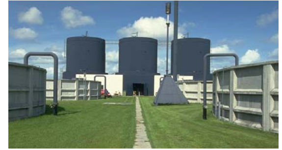
A modern Joint Biogas Plant
