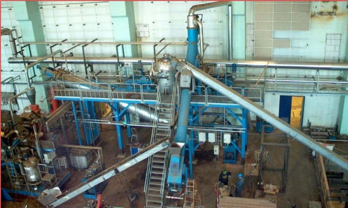
Inbicon pretreatment pilot plant
